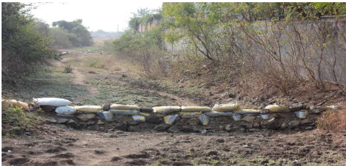
Canal constructed by NSS volunteers
