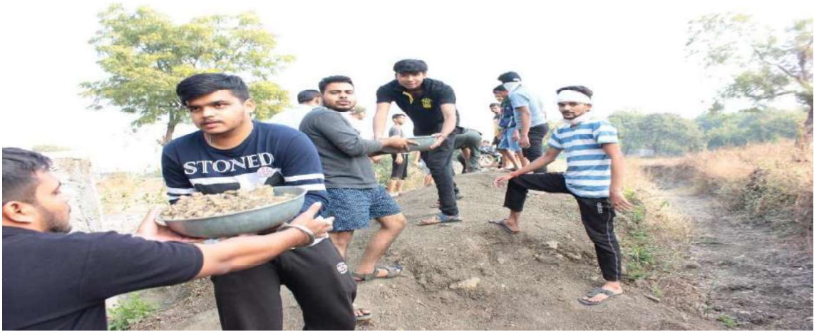
Students constructing canal
