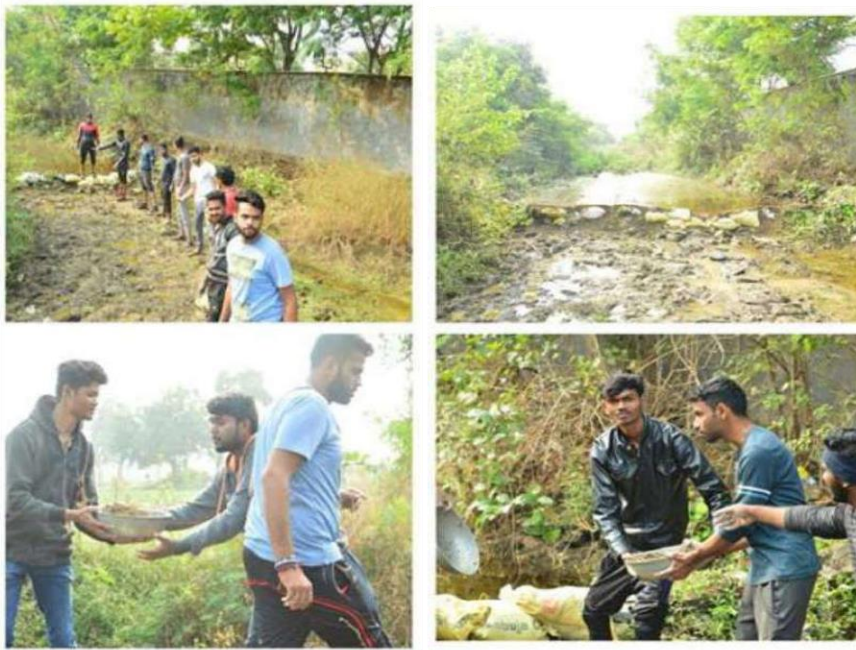
NSS volunteers constructed a small canal wall of rock and sand
