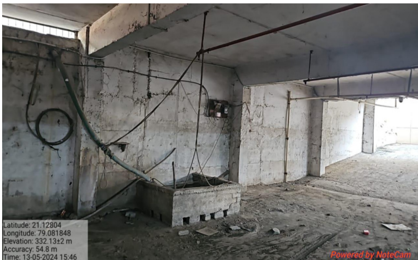
Chemicals from various department collected here in the separate tank and properly treated
