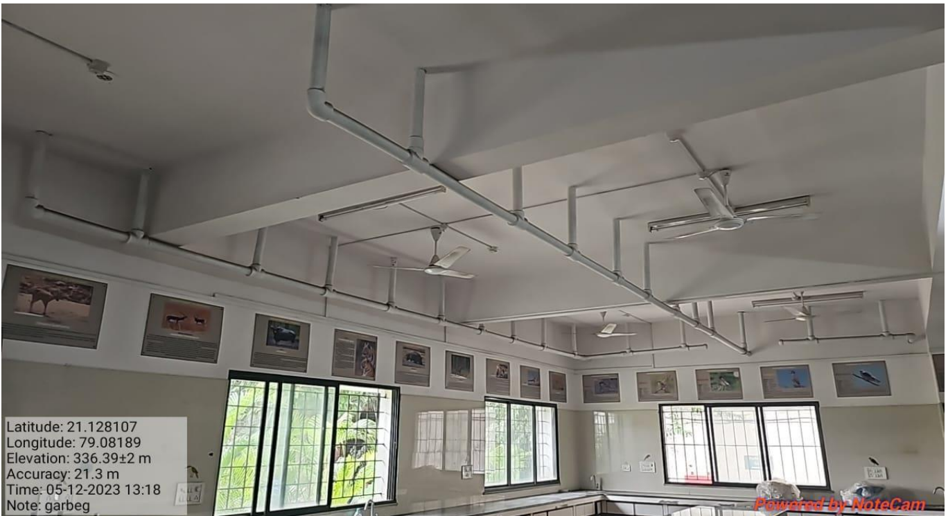
Waste chemical pipes connected with the chemical basins
