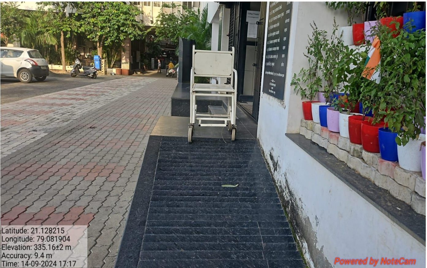
Ramp facility in block C
