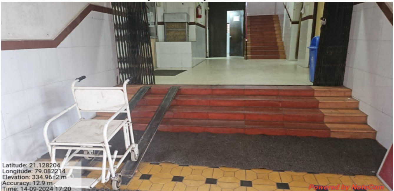
Ramp facility in block B
