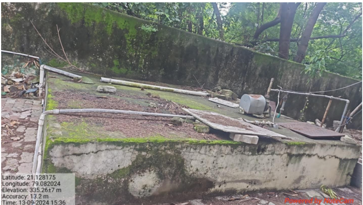
Construction of Bunds and Tanks
