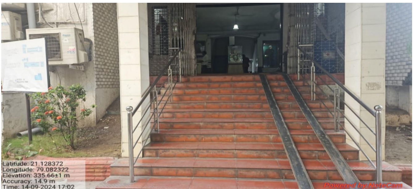
Ramp facility in block A
