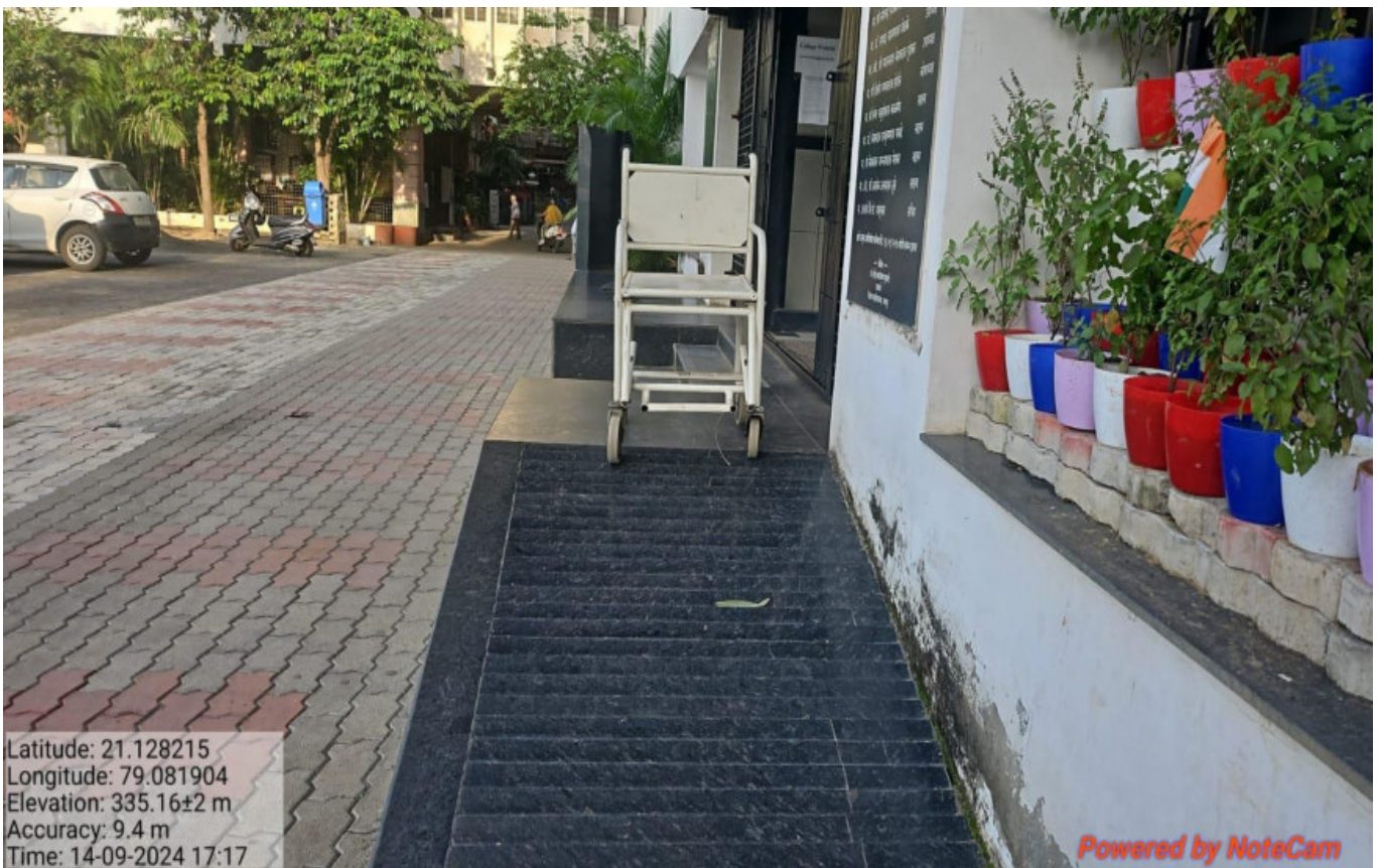
Ramp facility in block C
